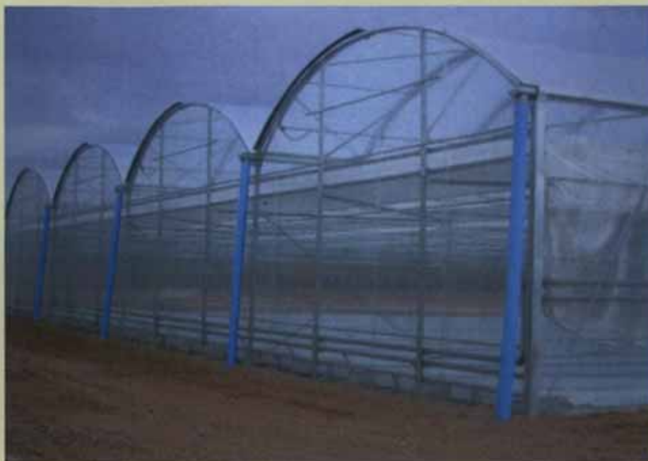
Frontal invernadero multitunel.
